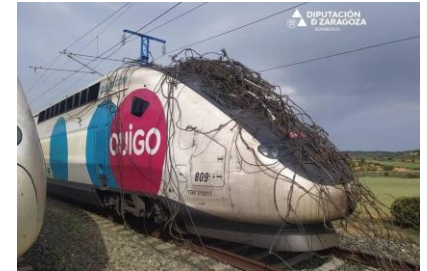
Contact between catenary and pantograph
